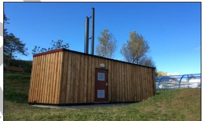
Ardrishaig Primary School biomass boilerhouse
