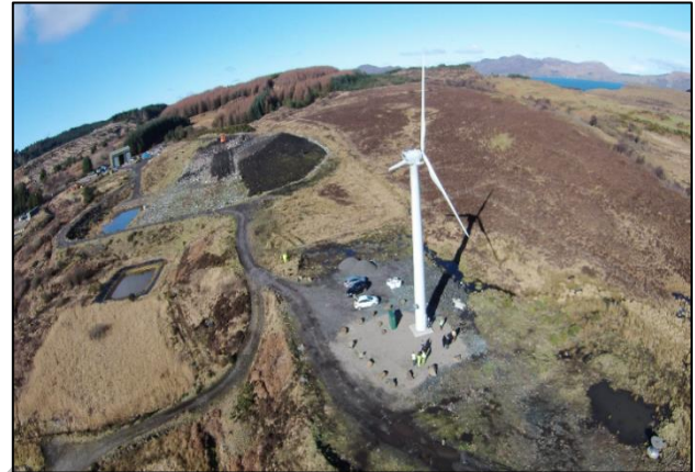
Council owned windturbine @ Glengorm Landfill, Mull
