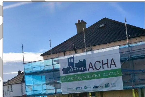
ACHA's External Wall Insulation works in Oban
